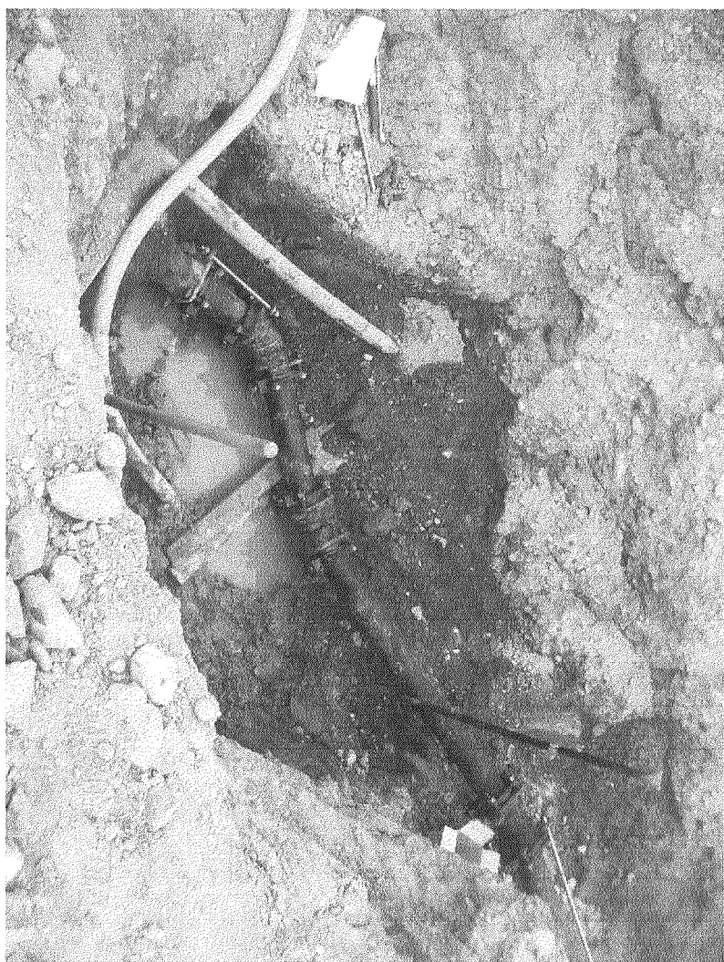
1 CONNECTION TO EX FIRE LINE NTS
